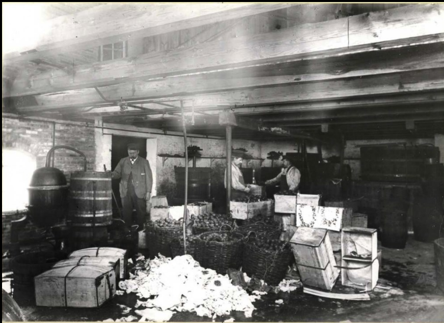
Views of the factory in Faaborg. The buildings were rebuilt into the art museum.
