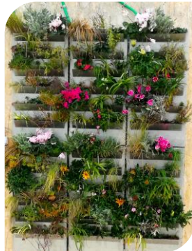
Greywater-fed facade panels with edible plants (alchemia-nova GmbH)
