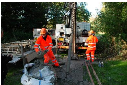
Figure 10: Investigations on soil conditions
