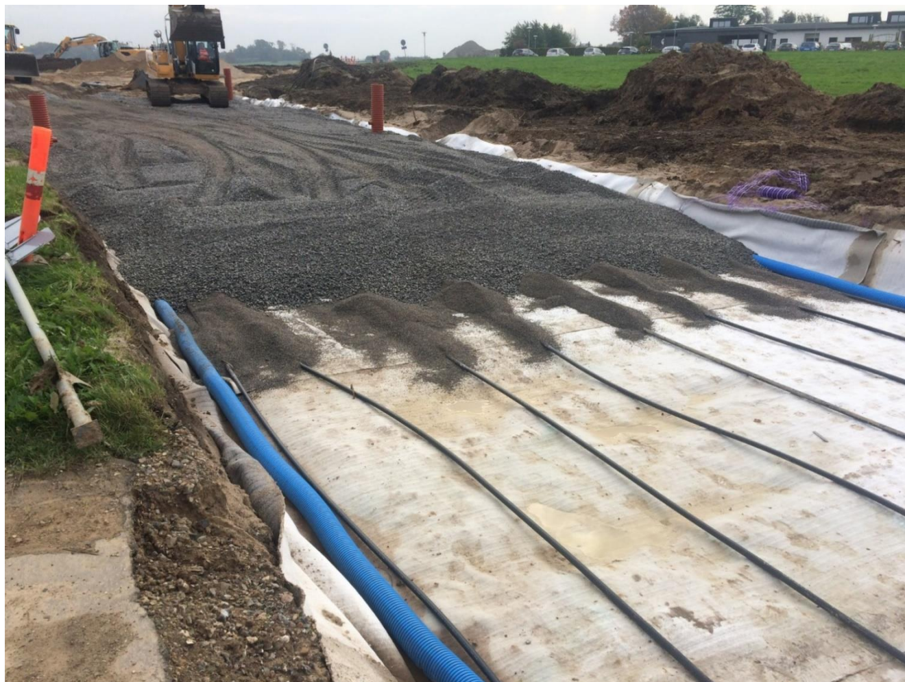
Figure 2. The construction pit with the bentonite membrane (white geotextile), blue Ø160 mm drainage pipes on the sides, and black geothermal piping loops embedded in soft DrænAF gravel with the coarser DrænStabil gravel on top. The kindergarten with the GSHP using the Climate Road as a collector is visible in the top right corner of the picture.
