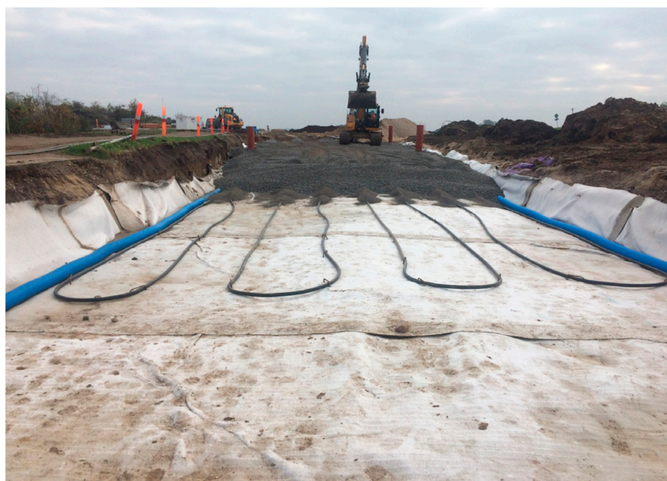
Figure 3. The Climate Road during construction.
