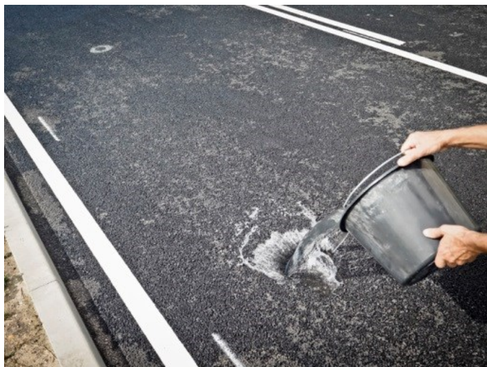
Figure 2. The water quickly disappears down the permeable asphalt of the climate road
